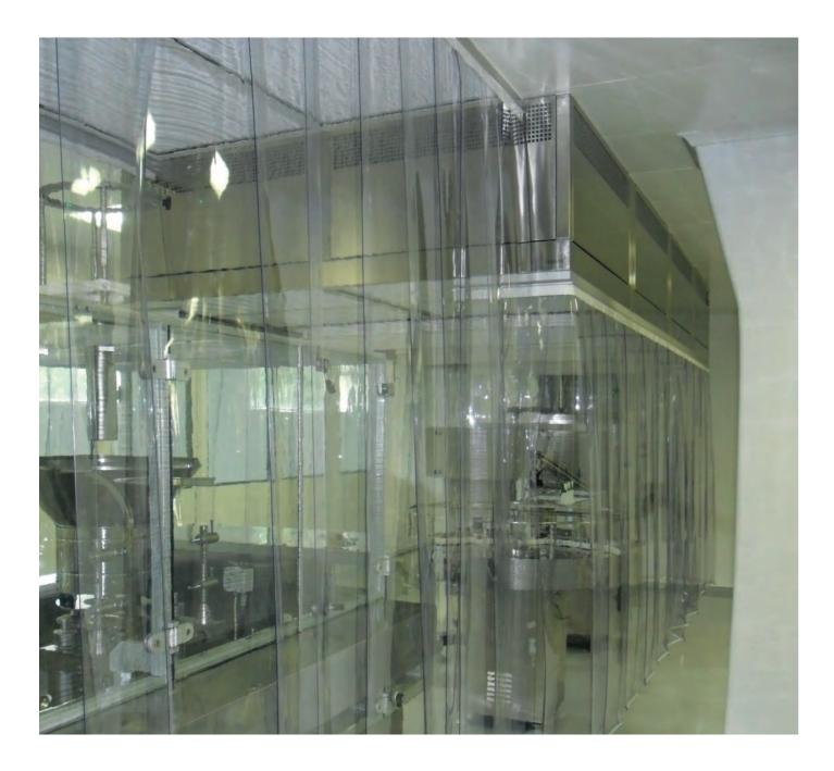
As a system supplier, clean-tek manufactures laminar flow modules that provide protection against airborne particles in a controlled production environment.
